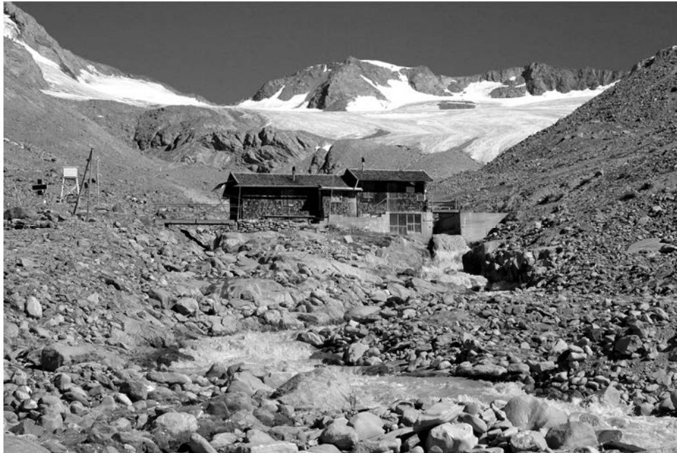
Figure 1: Pegelstation Vernagtbach situated at 2640 m a.s.l. with the climate station on the left. (Photo taken September 30, 2003).
